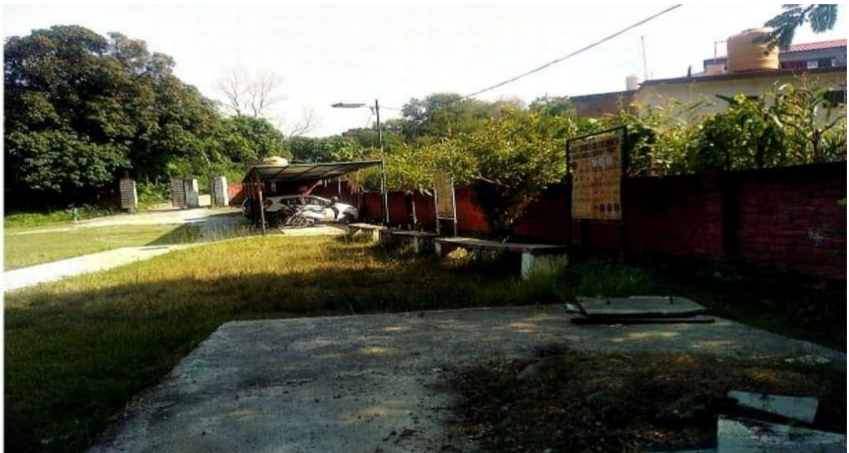
(Rain harvesting tank in GDC Dhaneta college campus)
